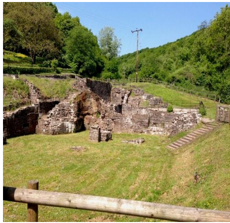
Tintern Abbey Furnace
